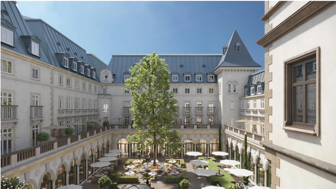
The Florentin Courtyard
